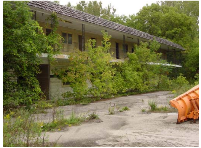
Former motel building at Flory Property in Center Rutland
